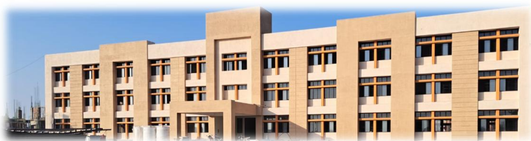
Building Under Construction
